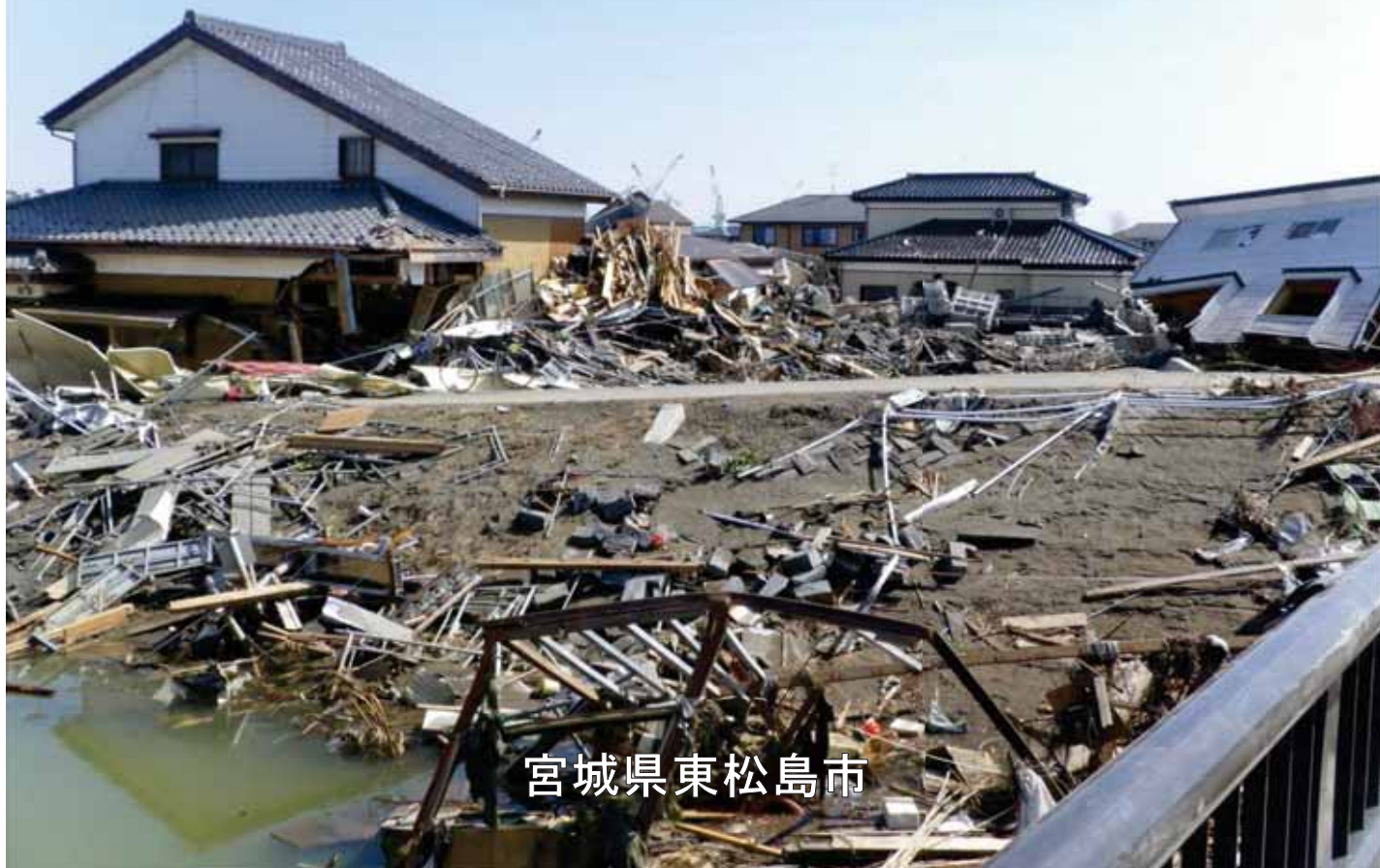
1016_2_018_020170_東松島市_2011.3.19_大曲浜_下浜橋
